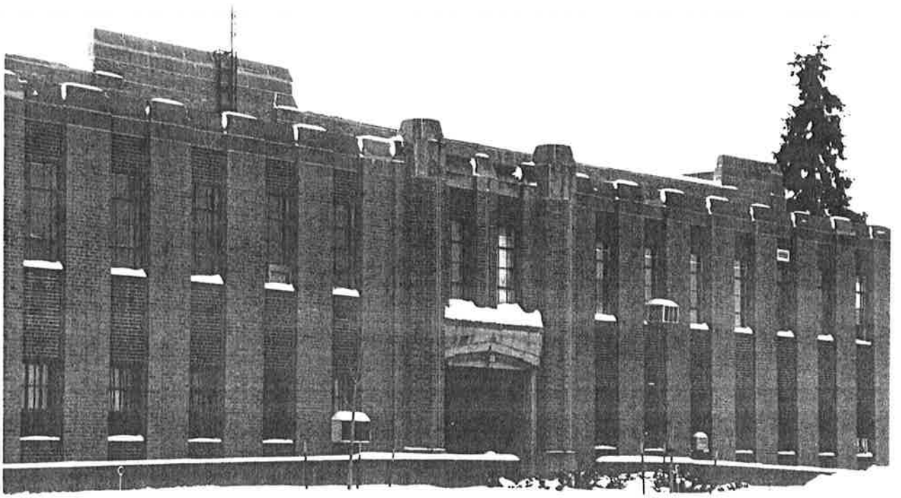
North-east facade looking west
