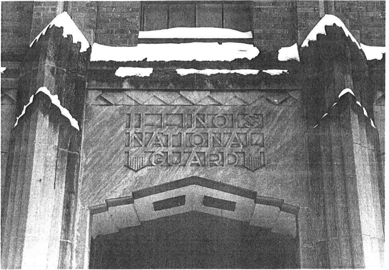
Front facade main level detail
